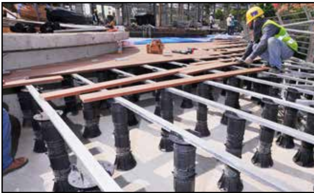
BlackJack provides stable support for installation of decking using joist holders
